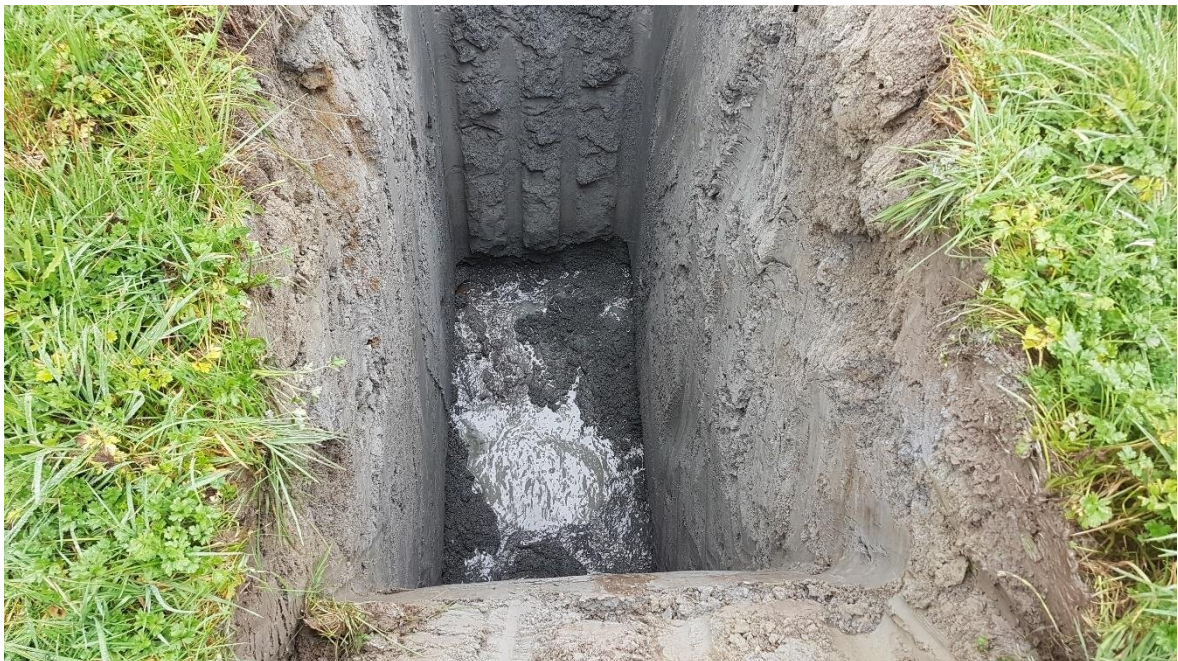
Figure 4. Photo of test pit 06
